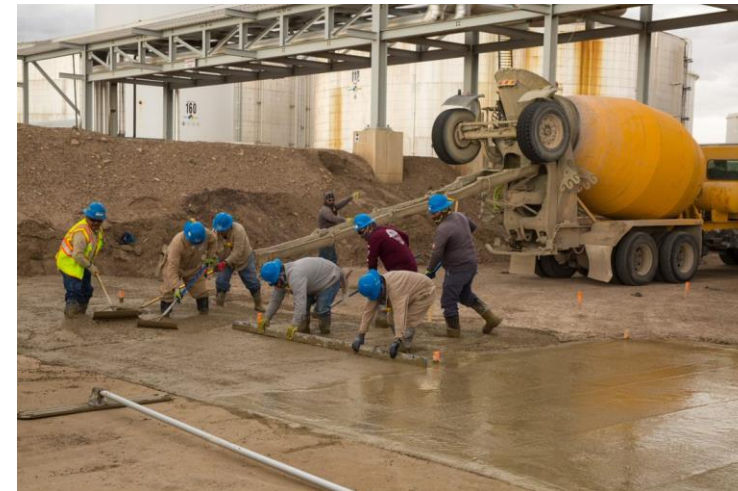
Leveling concrete for RD at Great Falls
