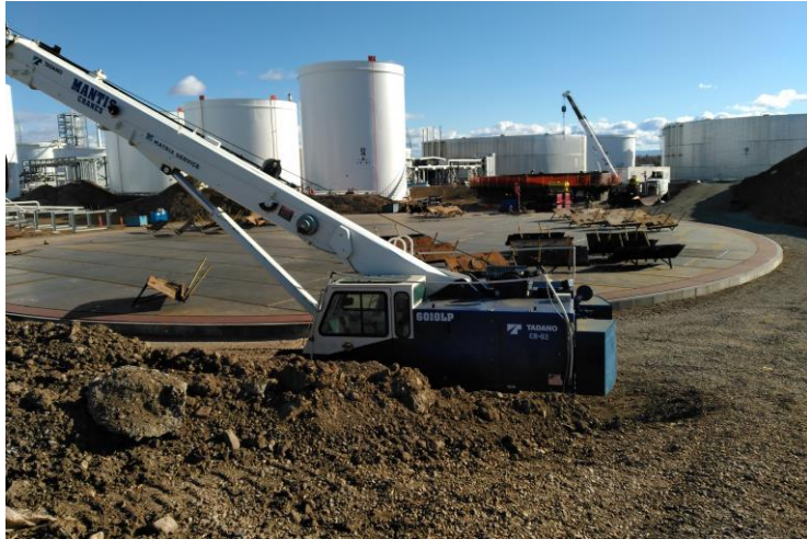
Crane activity on RD tank farm at Great Falls
