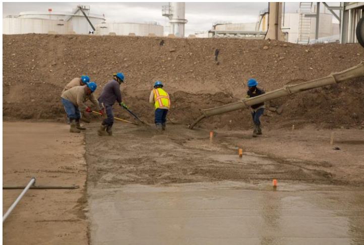
Pouring concrete for RD at Great Falls
