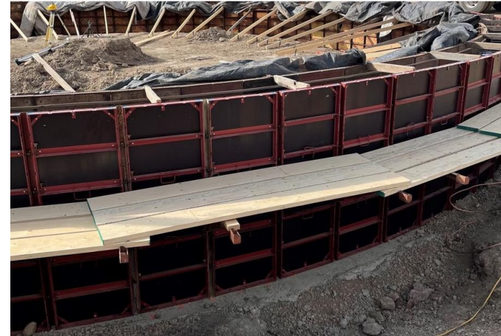
New RD tank construction at Great Falls
