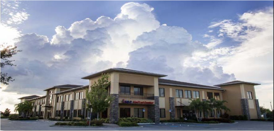
Parkway Professional Plaza Lakeland, FL (Tampa)
