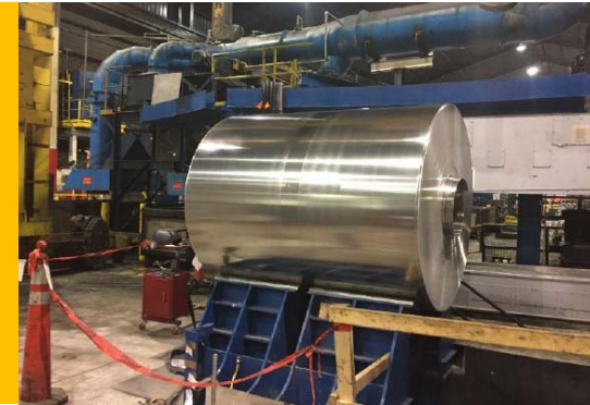
HOT MILL WIDENING & UPGRADE
