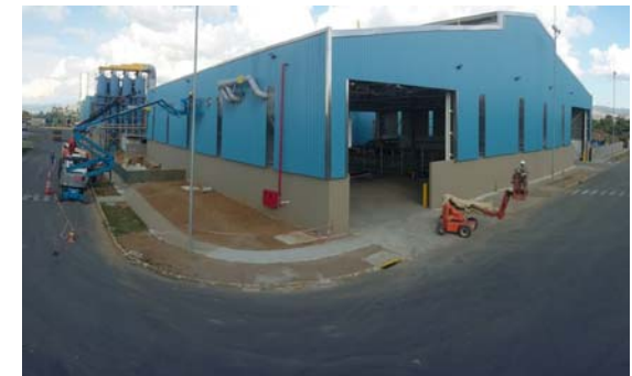
New dross house in Pinda, Brazil
