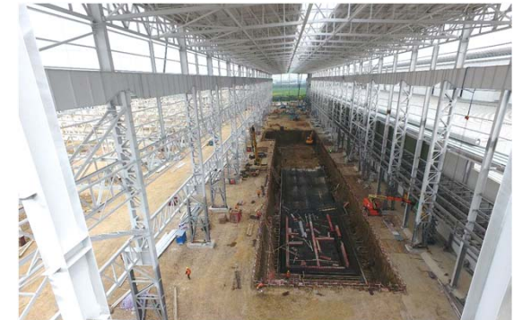
CASH line pit foundation in Changzhou, China
