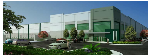
Prologis Cheyenne Distribution Center #3 163,800 SF
