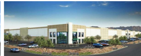
Prologis North 15 Freeway Distribution Center 410,600 SF
