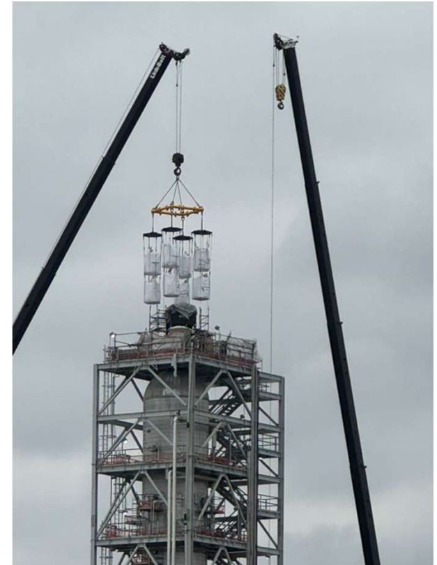
MaxSAF® 150 catalyst loading in April 2026
