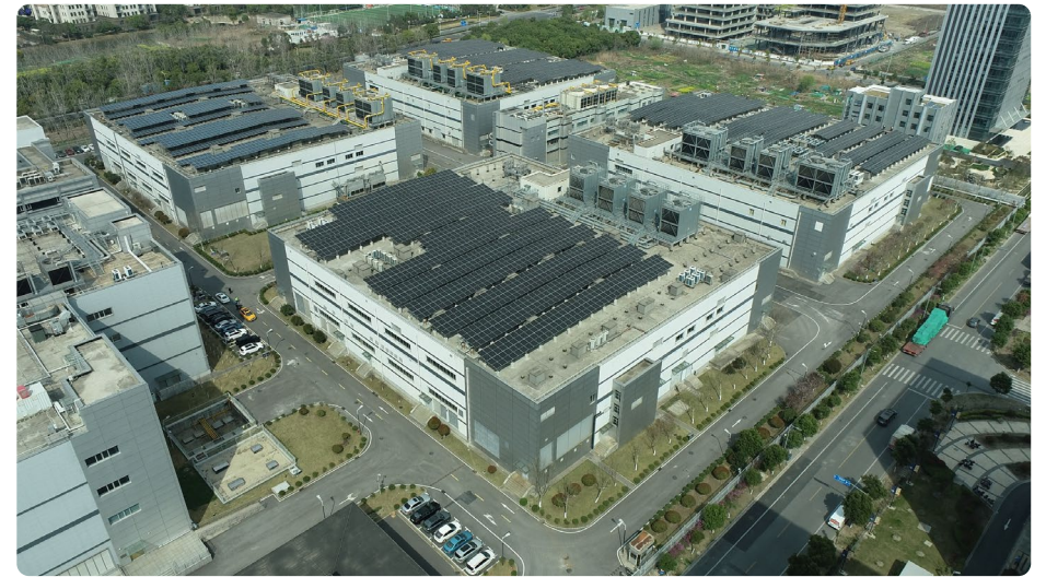
Tencent Shanghai Qingpu Data Center
