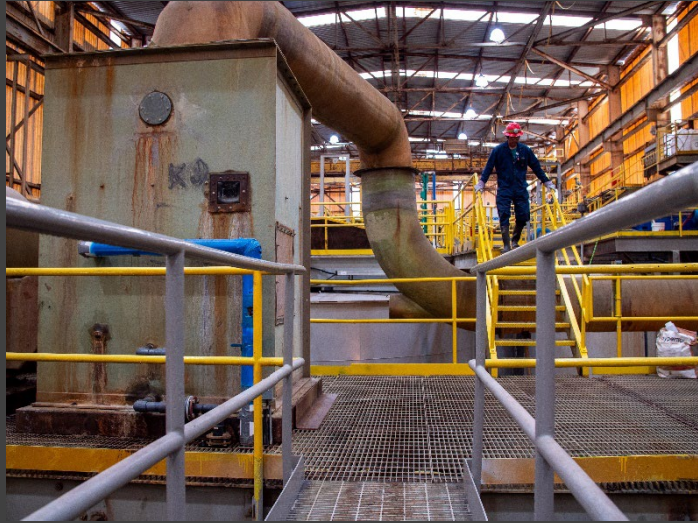
Worker inside of Energy Fuels' White Mesa Mill
