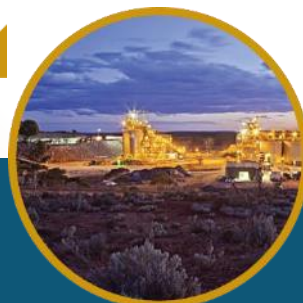
HGO mill fed at 100% capacity 1.4 Mtpa (4,000 tpd)
