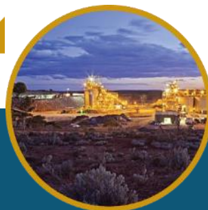
HGO mill fed at 100% capacity 1.4 Mtpa (4,000 tpd)
