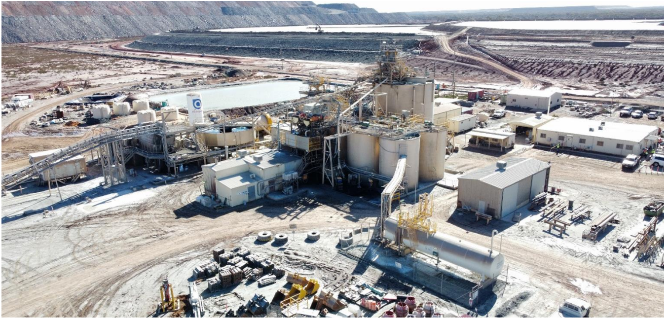
Figure 1: Lakewood Processing Facility Ariel Photo (July 2022)
