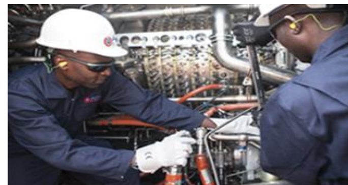
Pictured: APR personnel maintaining an aeroderivative turbine
