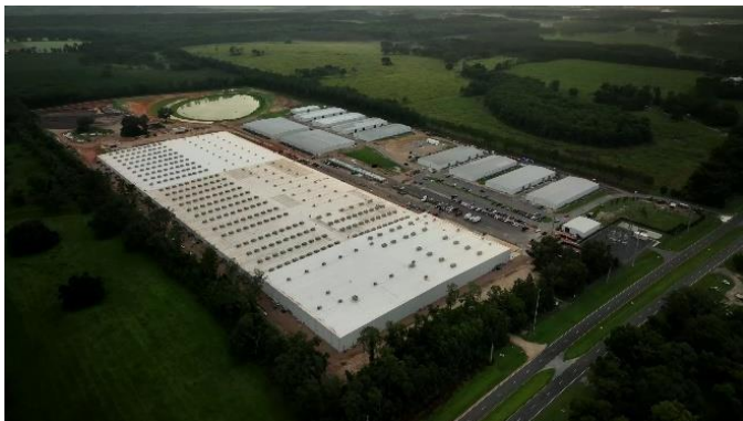
Our Jefferson County, FL cultivation facility, one of the largest and most sophisticated in the world, produces consistent high-quality flower at industry-leading scale.
